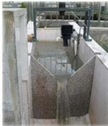
Installation of stilling well
